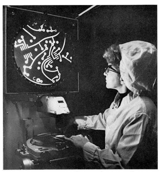
OPTICAL COMPARATOR with 100 magnification is used by Dorcas Gabaldon (4233-3) to check for possible breaks or flaws in circuit paths.
